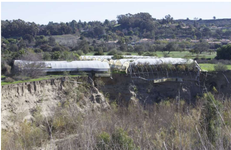
A nursery greenhouse perches precariously atop an eroded bluff along Oso Creek in southern Orange County. The SMC has played a key role in helping stormwater managers rethink how legacy flood-control BMPs can be used to both guard against the destructive effects of erosion and other landscape alterations, and simultaneously still protect property and humans from flooding.
