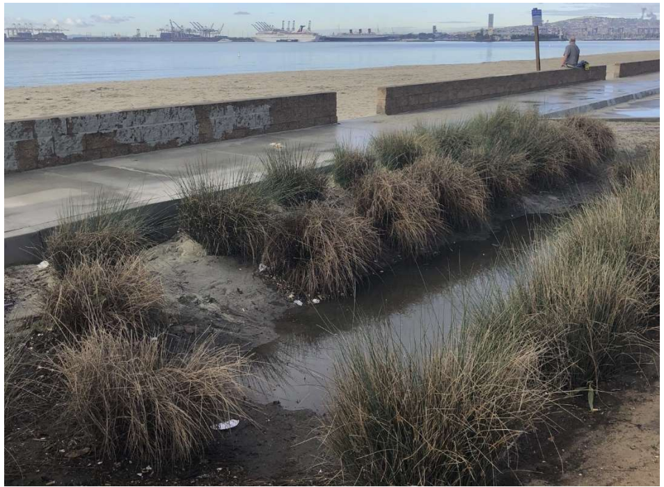
A bioretention BMP that abuts the shoreline in Long Beach filters and removes stormwater contaminants, helping to protect beach water quality. The SMC has been working to generate Southern California-specific data on the performance of these and other types of BMPs in an effort to optimize their ability to treat and remove pollution in runoff.
