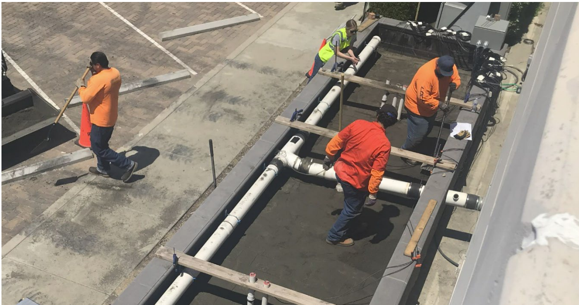
A field crew installs monitoring instruments and engineered media in a bioretention BMP in Riverside County. Microplastics researchers are using an SMC-developed network of BMP monitoring sites across southern California, including the one above, to investigate the degree to which BMPs can remove microplastic contamination in runoff. Photo credit: Adrian Montoya, Riverside County Flood Control and Watershed Protection District
