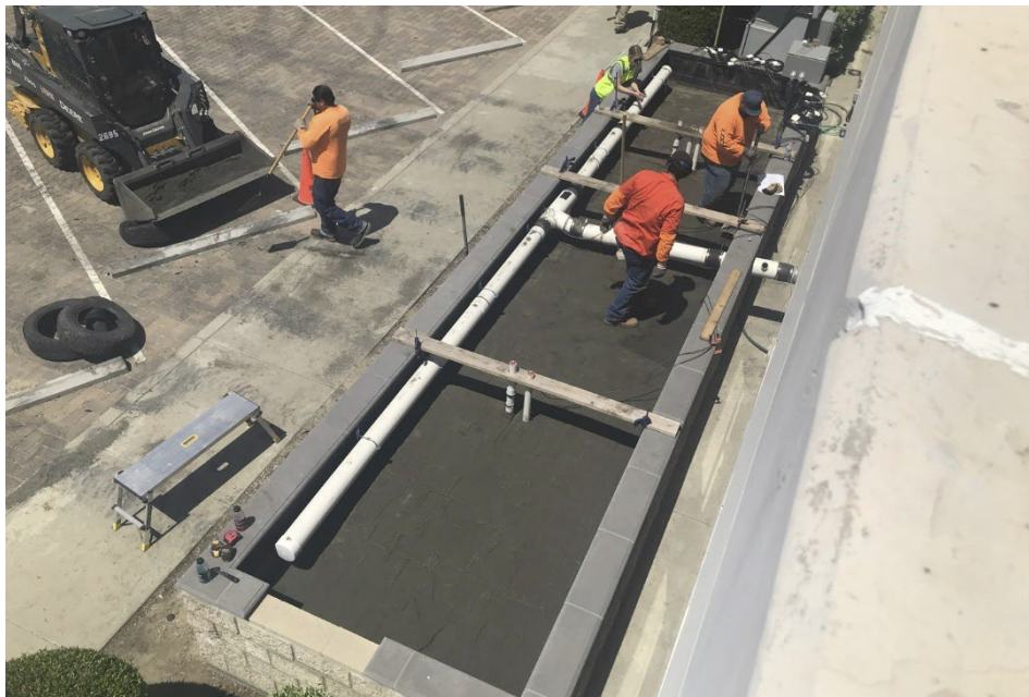
A field crew installs monitoring instruments and engineered media in a bioretention BMP in Riverside County. The site is part of the SMC's new Regional BMP Monitoring Network, a network of southern California stormwater BMP sites completed in 2024 to generate high-quality, comparable data sets quantifying the performance effectiveness of structural BMPs.
